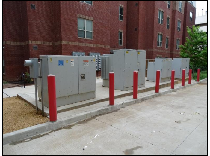
2. Main electrical transformers
